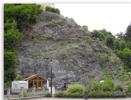
Rock face after nailing
