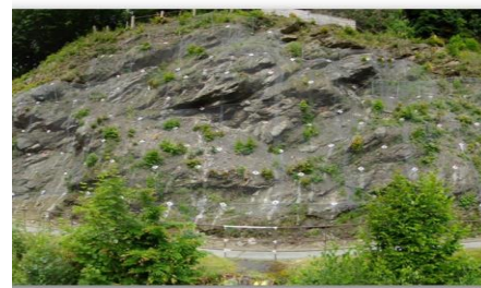
secured rock face
